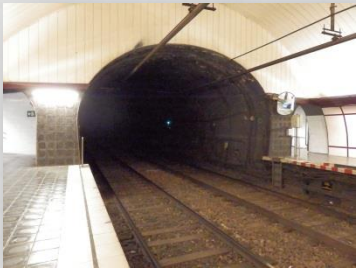
one wide tunnel with two rail tracks without middle wall
