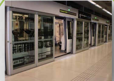
a single tunnel with one rail track separated from the platform by a wall with mechanical doors (platform screen door systems)
