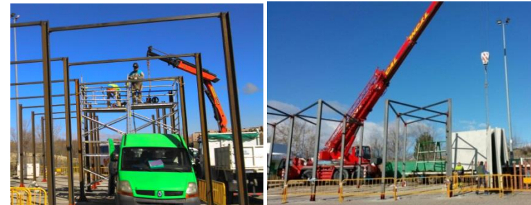
Construction of double street canyon
